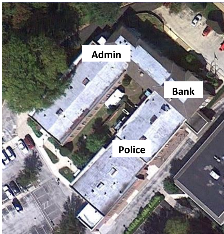
Figure 1: Whitemarsh Township Building, Aerial View (© 2013 Google Earth)
